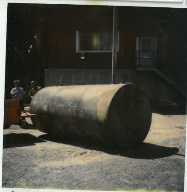
8-25-82 Removal of 12' tank at Power Plant
